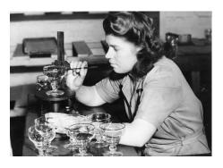
This lady is applying gold lines to wine glasses, using a brush to paint thin lines of liquid gold suspension, which was then fired on in a kiln. Do you think you have a steady enough hand to do her job?
